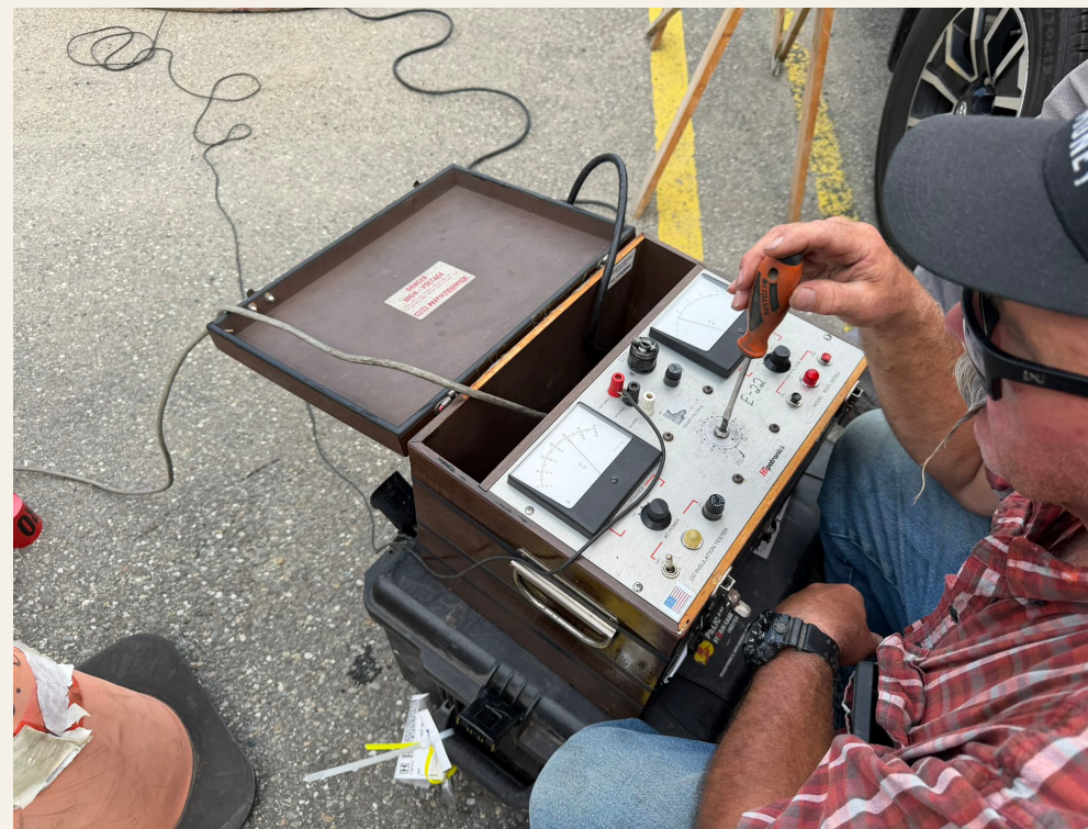
Final test of full cable length - very low leakage!
