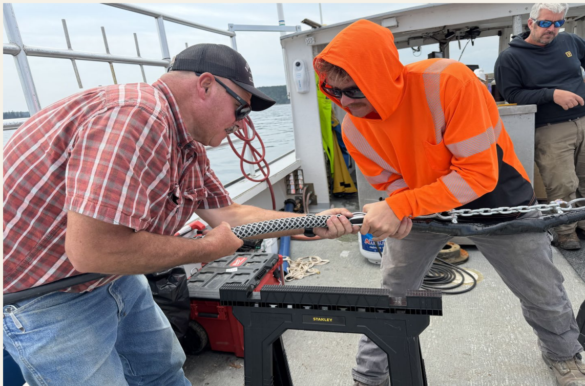
Splicers add tension protection on the final splice
